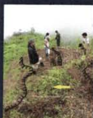
b) Presence of tension cracks
