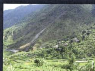
d) Emergence of springs, seeps, or saturated ground in areas that have not typically been wet before
