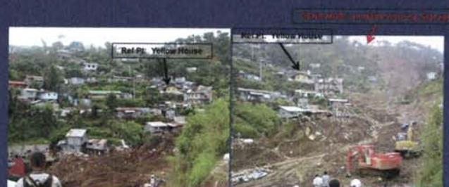
AFTER Typhoon Pepeng, October 2009. Little Kibungan, Pugaos, La Trinidad, Benguet. Slopes bounding the southern portion of the area where debris slide. Also shown are large tension cracks developing upslope, near the crown of the slide that hit Sitio Little Kibungan.
